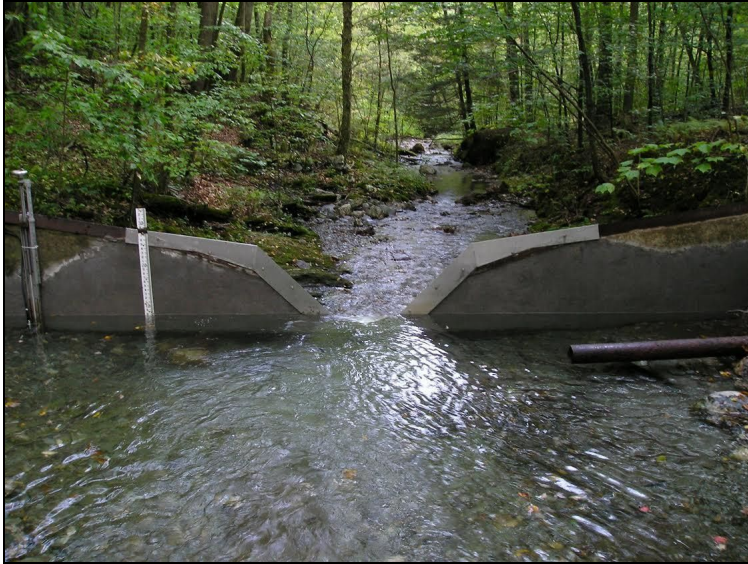
Figure 3. Birch Brook weir, looking downstream. Volume flux (discharge) of water has been measured continuously since 1985 using pressure transducers.
